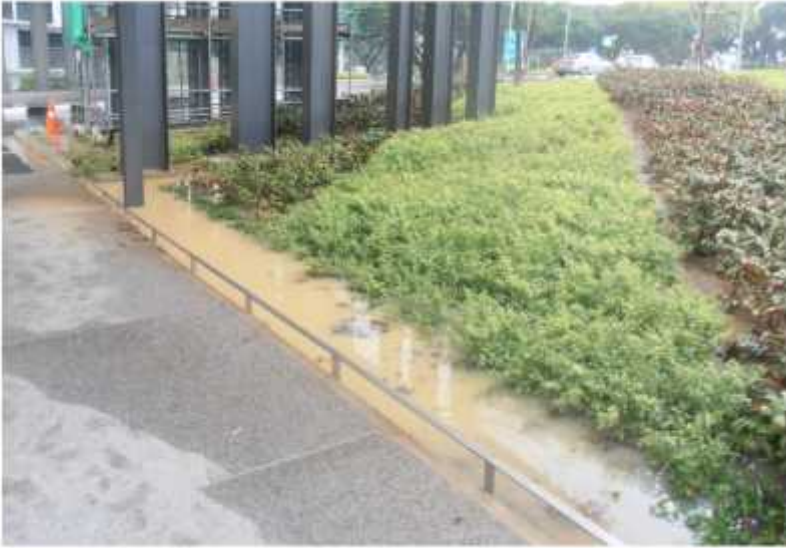
Figure 12.3 Poor drainage
