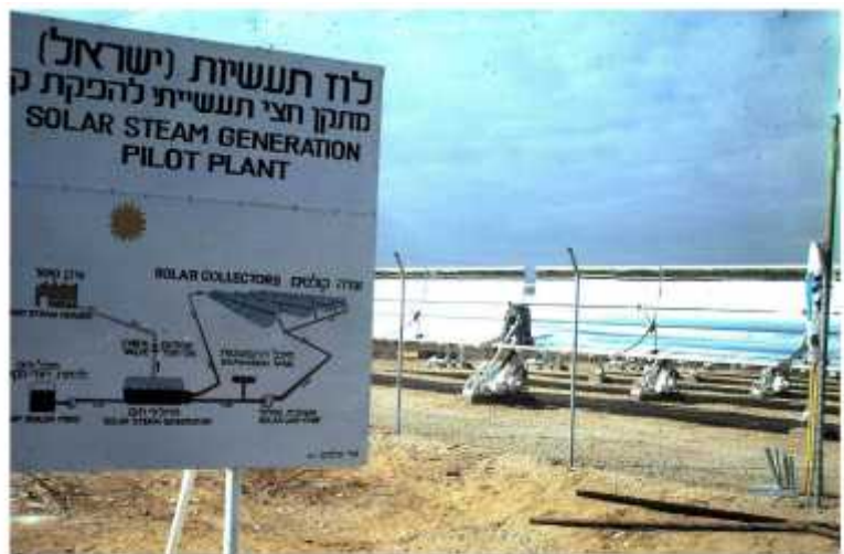
Figure 6.4 Part of the LuZ SEGS-1 Solar Array
