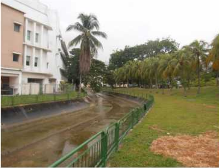
Figure 7.5 Section of urban drainage system
