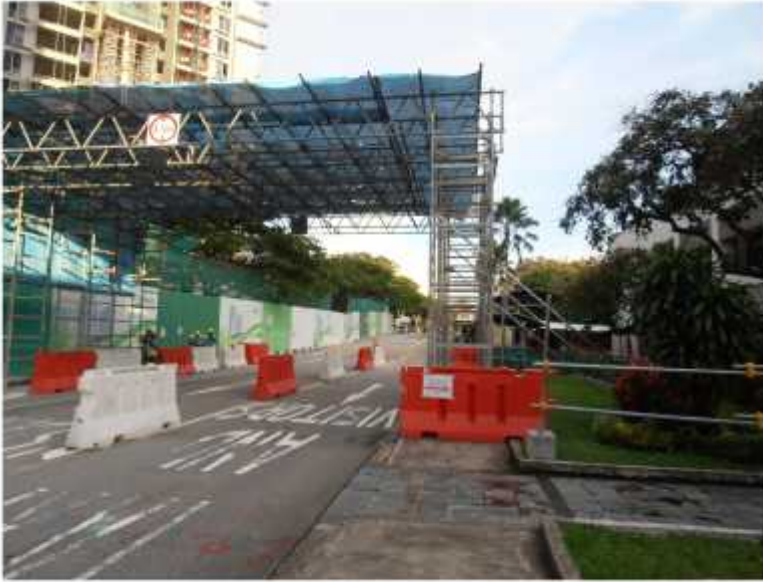
Figure 9.16 Temporary diversion for pedestrians
